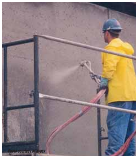
Sprayed on surface application.
