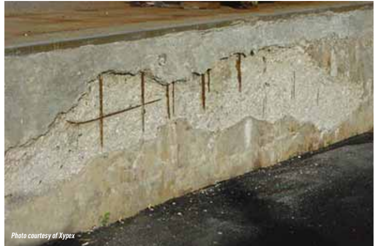
Example of concrete deterioration caused rusting of the reinforcing steel.
